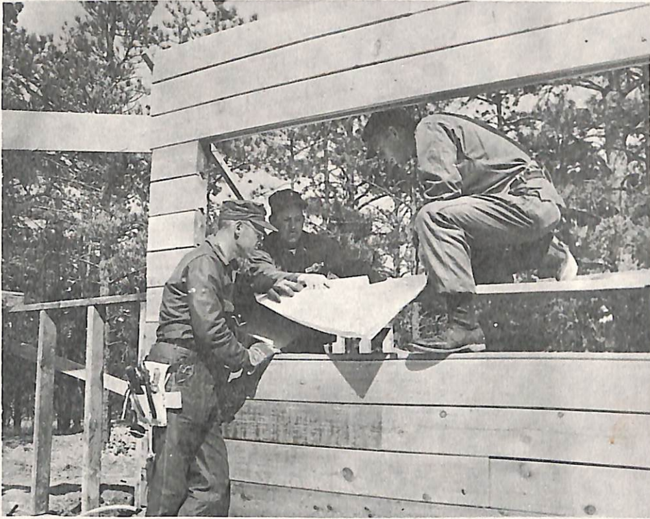
DINING HALL UNDER CONSTRUCTION
